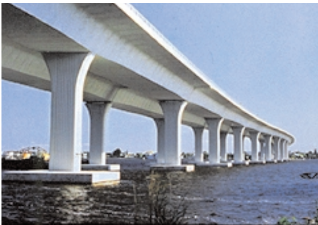
Fig. 1-34. Concrete bridges in seawater exposure must be specially designed for durability. (68667)
