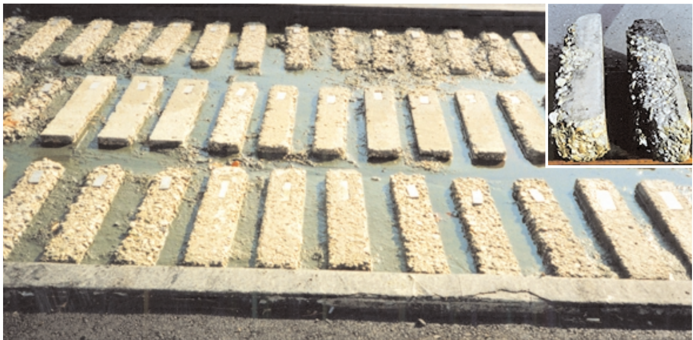
Fig. 1-32. Concrete beams after seven years of exposure to sulfate-rich wet soil in a Sacramento, California, test plot. The beams in better condition have low water-cementitious materials ratios, and most have sulfate resistant cement. The inset shows two of the beams tipped on their side to expose decreasing levels of deterioration with depth and moisture level. (66900, 58499)
